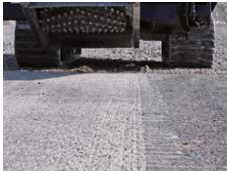
Multi-teeth drum for microplaning + line removal
