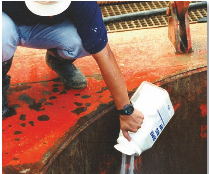
Mixing Directly into the Excavation
