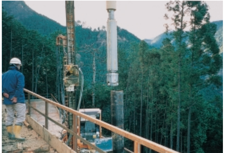
Piling After casing through the collapsing overburden, insert a H-steel, then pull up the casing.
