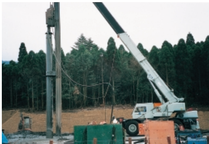
Geothermal · Oil Well Surface drilling down to 50m in depth for geothermal and oil well.
