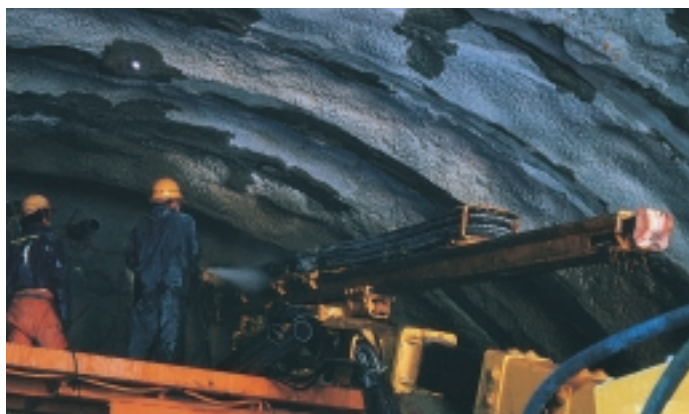
Fore Piling For piling as a reinforced method of tunneling in collapsing overburden.
